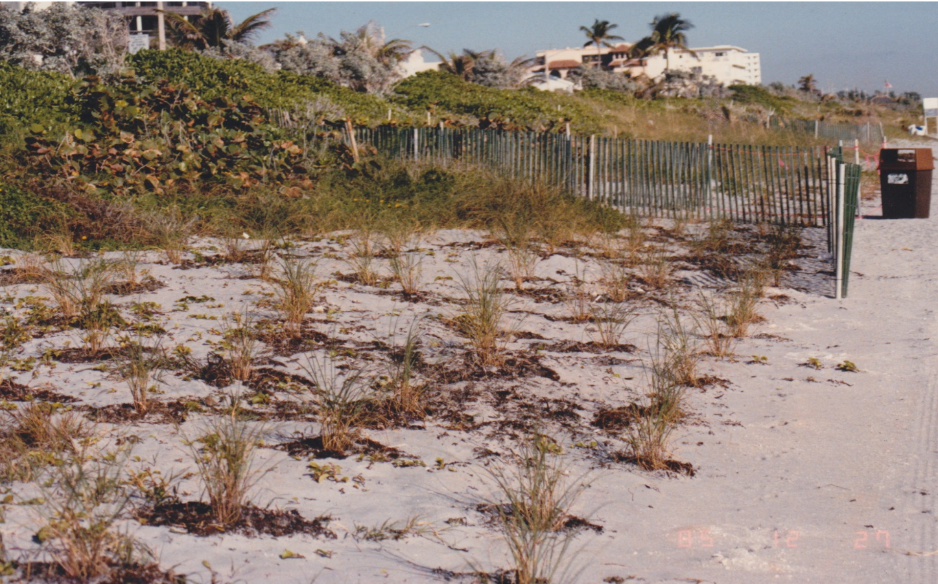
1985 dune planting installed sea oats in a 6 to 12 foot wide Strip just to seaward of the exotic Hawaiian seagrape
